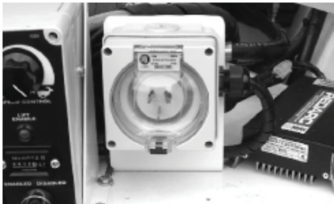
Figure 11.8 - Mains Power Connection For Charger
