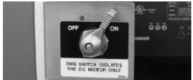
Figure 11.3 - DC Motor Battery Isolate Switch
