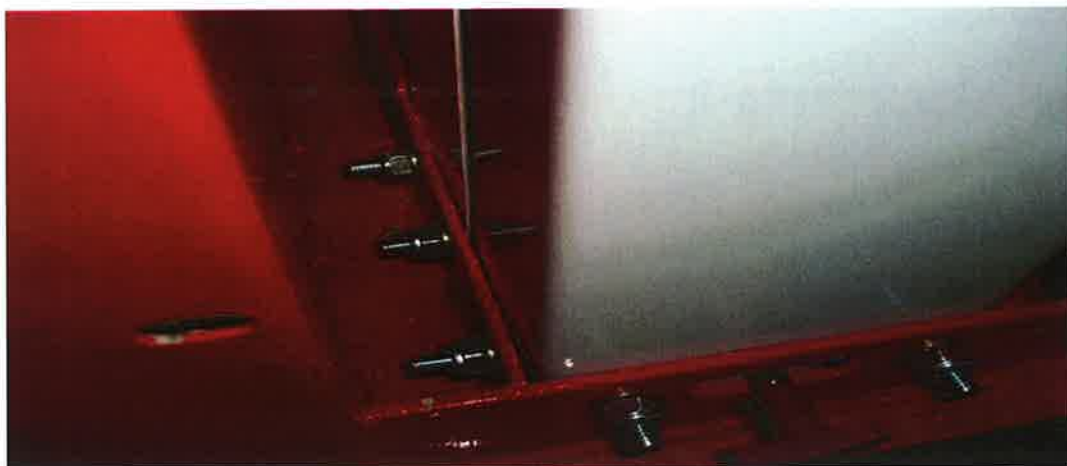
Fig.2 Location of left hand mast bolts. Note the one at the rear does not get changed.
