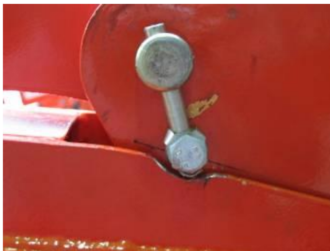
Fig 3 - Upper Boom ground away to provide clearance.
